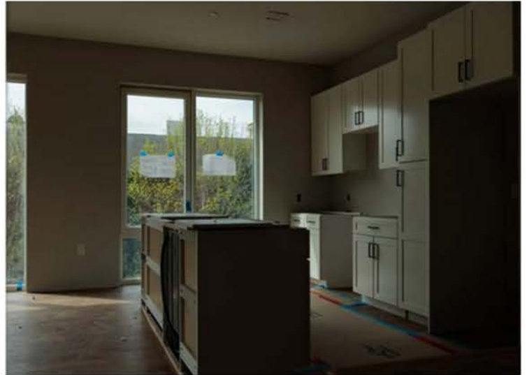
A kitchen under construction in one of the residential units.
